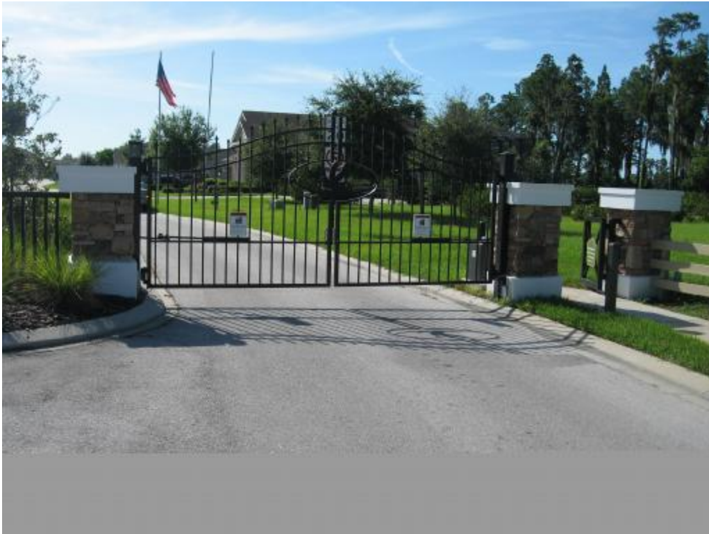
Vehicular Access Control
