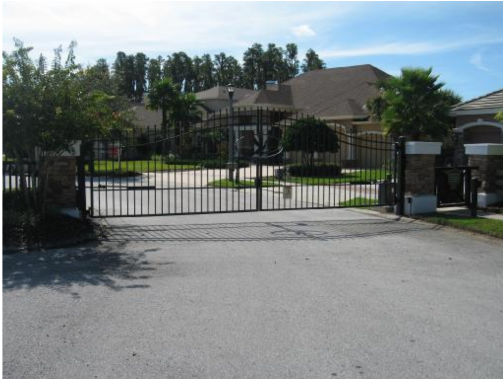
Vehicular Access Control
